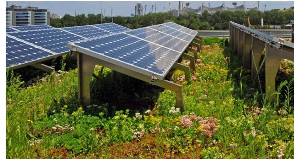
Biosolar roofs in study (photovoltaic + green)
